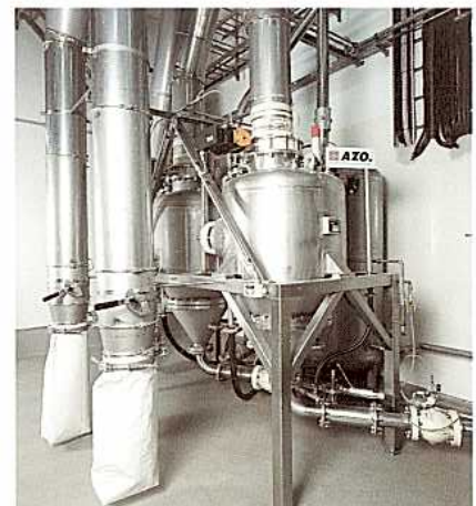
Pressure vessels for conveying heat-sensitive bulk materials
