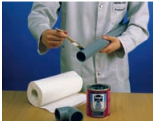
Applying the cement
