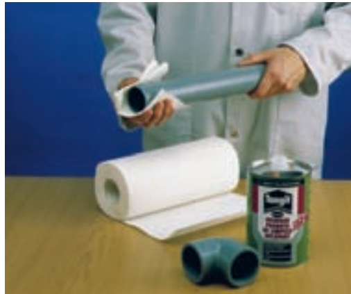
Cleaning the pipe and socket
