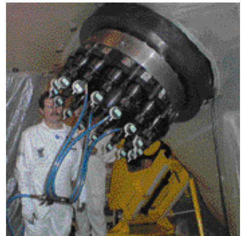
On-site intervention, tightening the man hole hatch on the primary cooling system of a steam generator.
