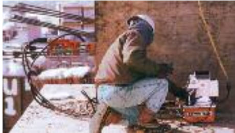
The PE60 used for pre-stressing.
