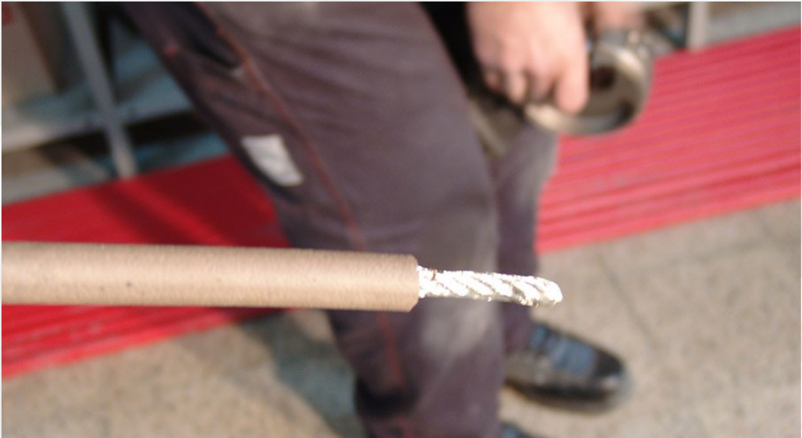
Application of the cable lug
