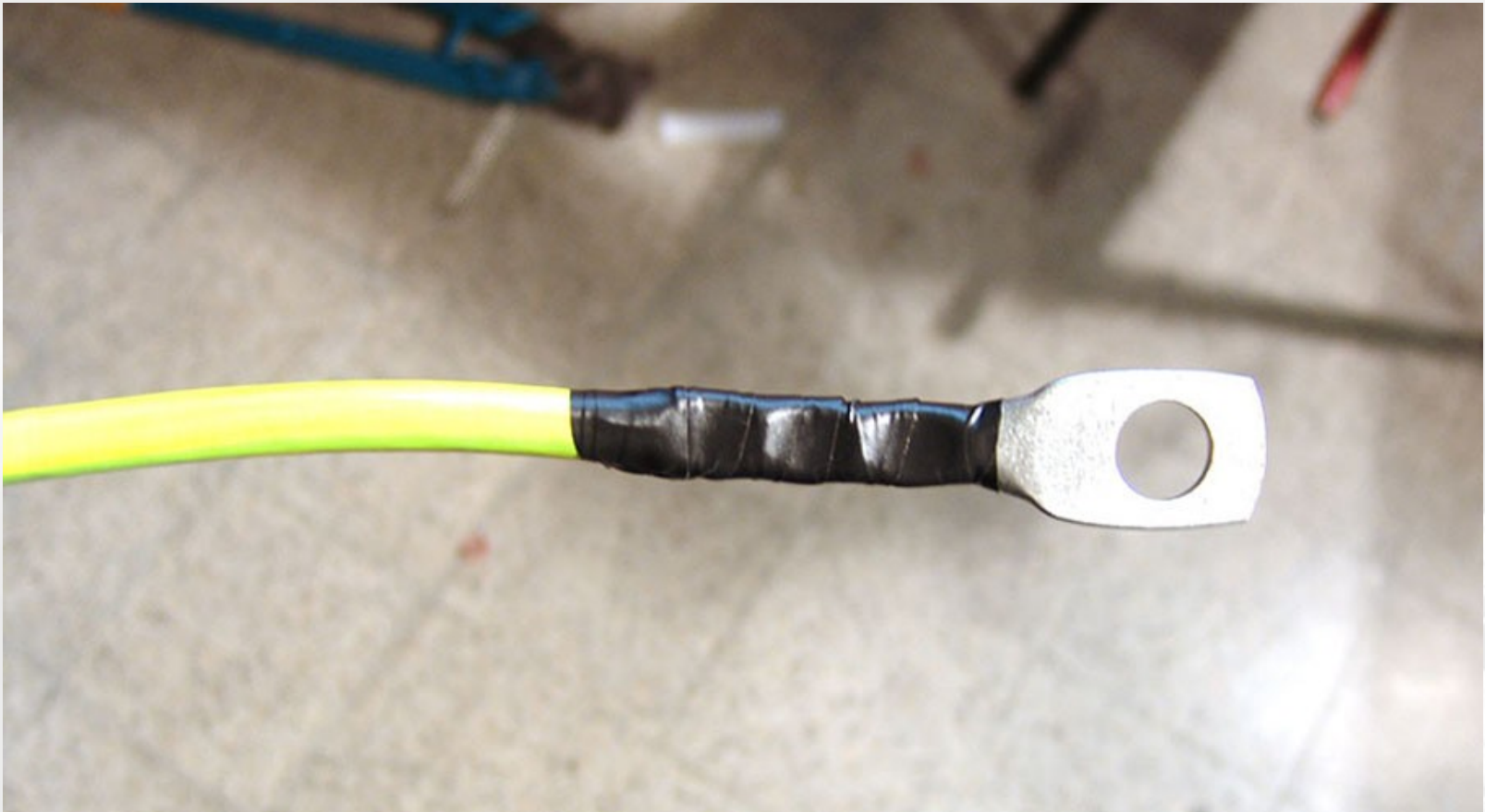
Application of cable lugs
