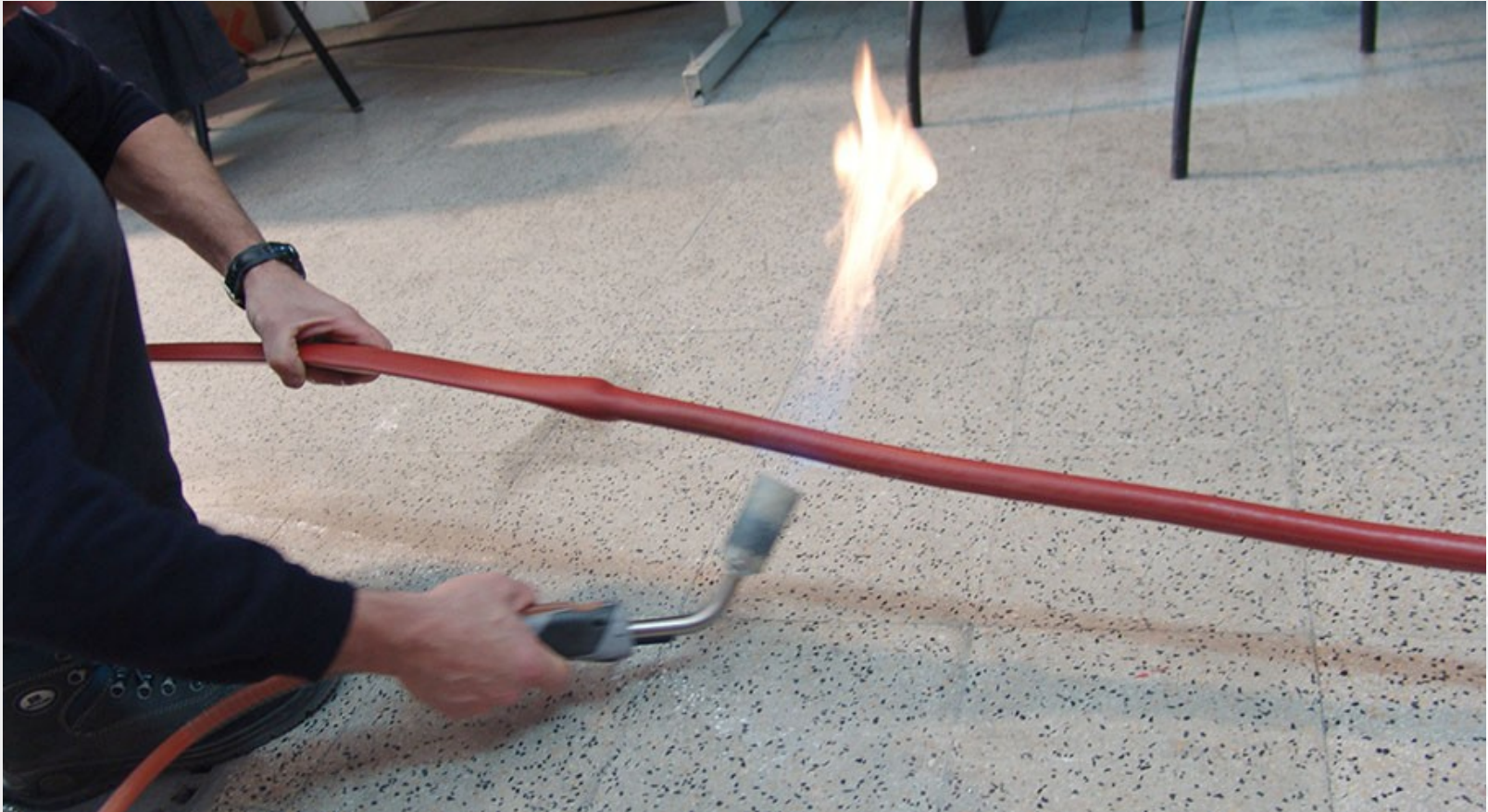
Application of heat shrinkable anti-tracking tube over the braid
