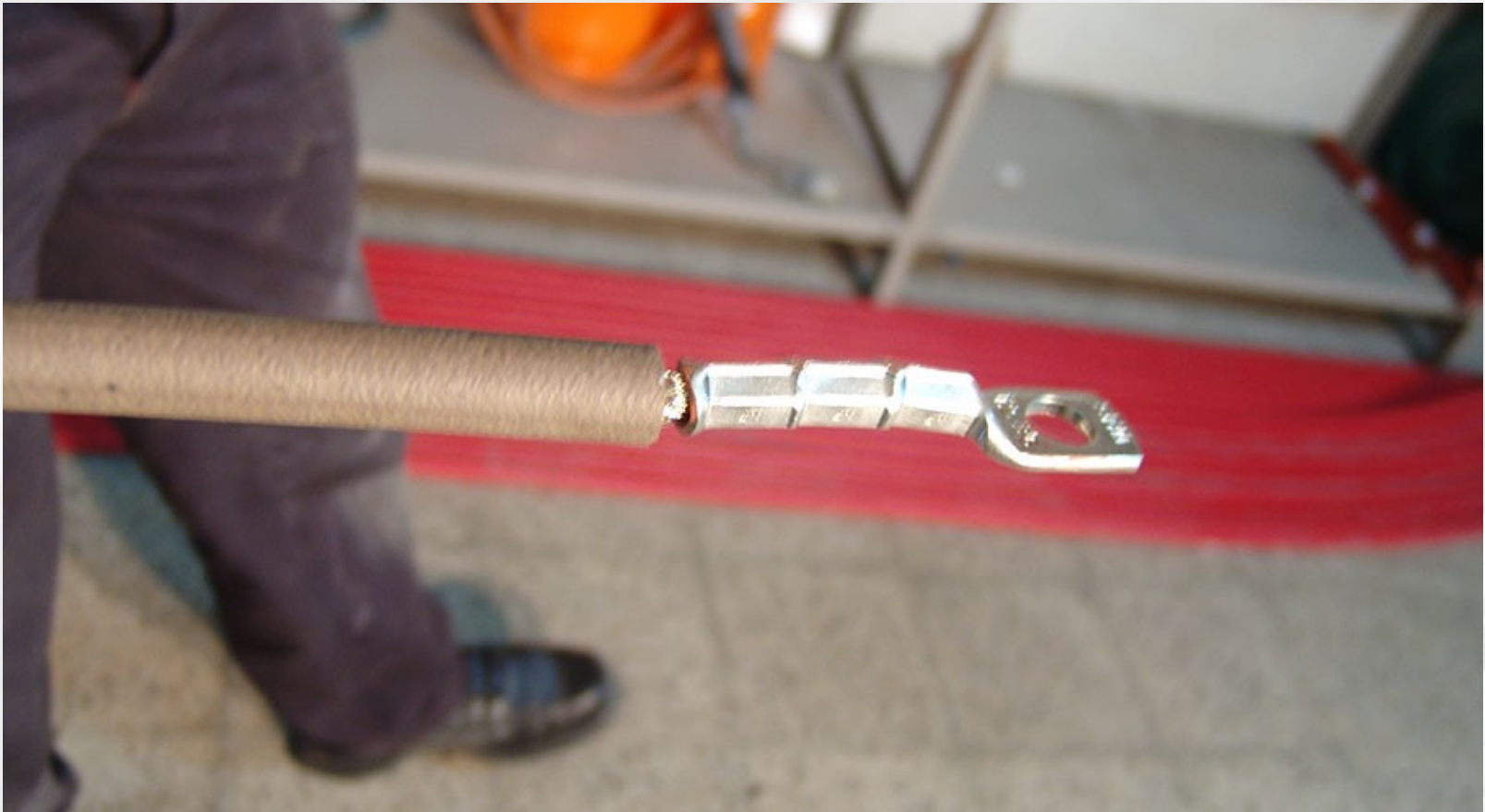
Application of the cable lug
