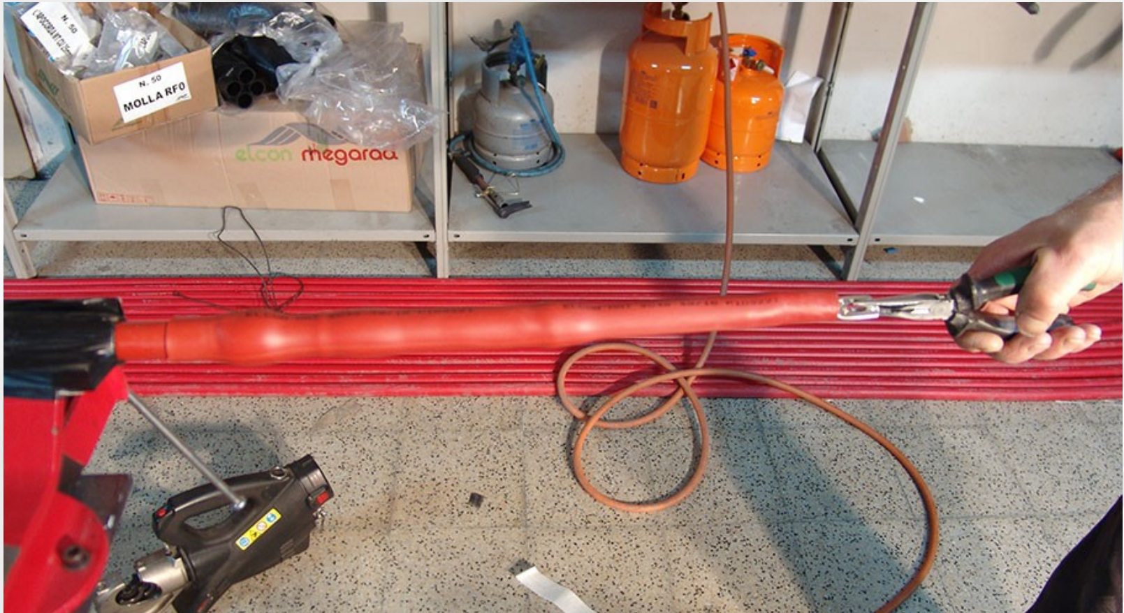
Application of the heat shrinkable medium voltage termination
