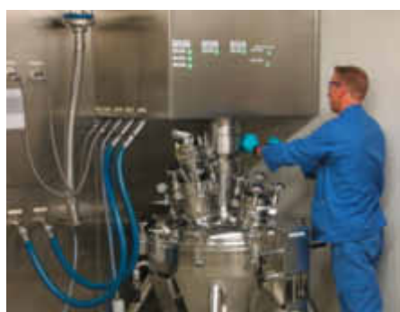
Connecting to drying station
