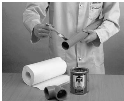
Applying the cement
